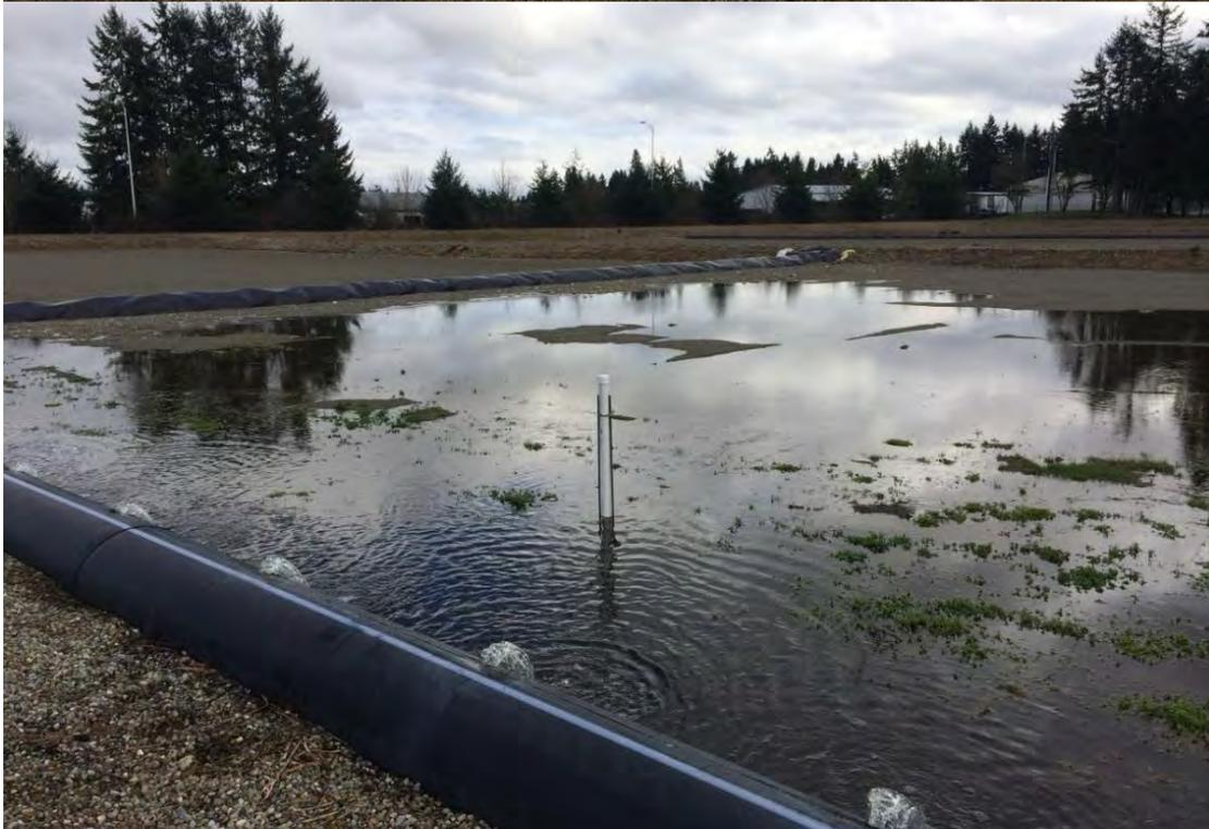
**Figure 3-2. Photograph of west side of Basin 4 during March 3, 2014, start-up monitoring with recharge flow rates  $\sim 0.7$  mgd.**
