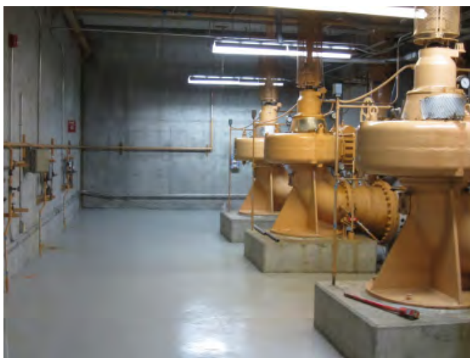
Figure 3-10. Influent pump volutes (two levels below grade)
