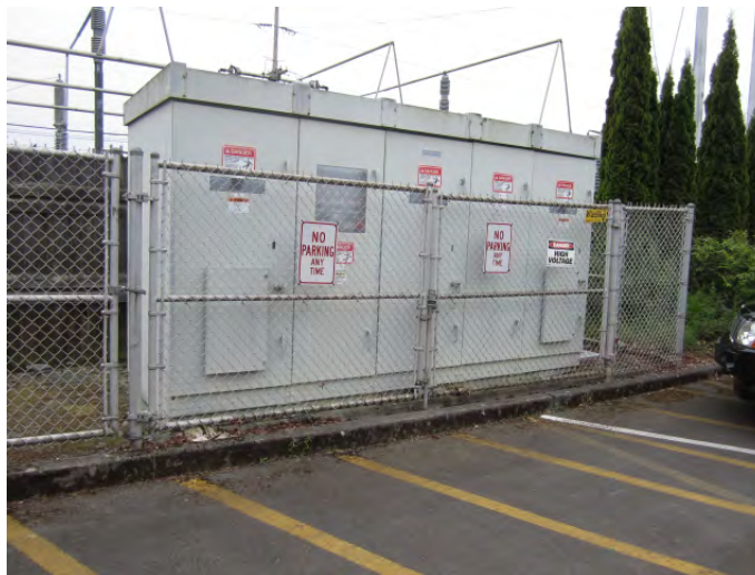
Figure 3-20. Service entry switchgear
