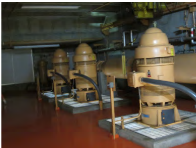
Figure 3-8. Influent pump motors (one level below grade)
