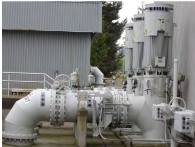
Figure 3-16. Outdoor effluent pumps
