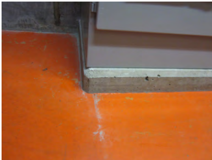
Figure 3-7. Electrical panel slab
