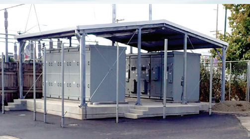
The switchgear project, completed in 2016, raised the electrical substation elevation by 1.5 feet and included watertight connections and enclosures.
