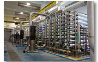
Reverse Osmosis (membrane, physical separation)
