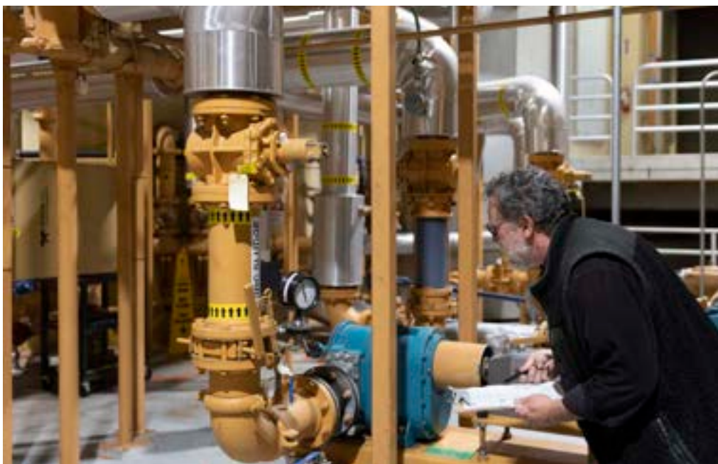
The Digester System Improvements project includes refurbishment of aging components associated with the sludge digestion system.
