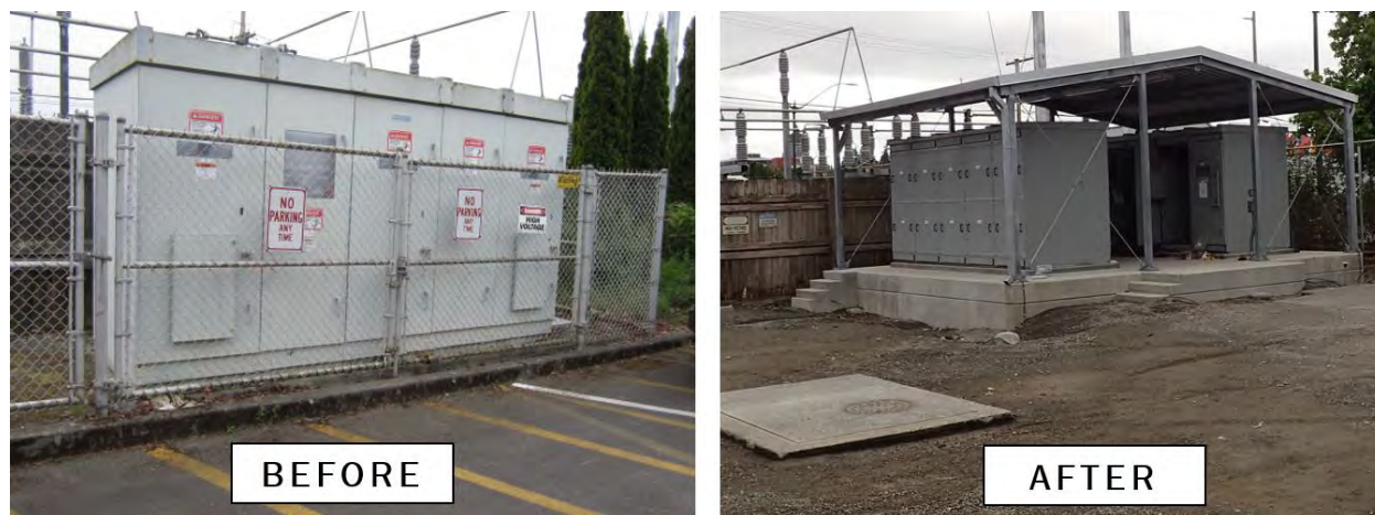
Figure 5-2. Renovation of electrical switchgear with elevated pad to reduce flooding risk
