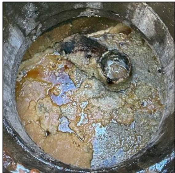
Inlet baffle first compartment
