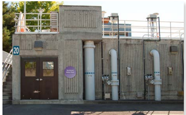
The Budd Inlet Reclaimed Water Plant uses sand filter technology to produce about 1.5 mgd of Class A reclaimed water.
