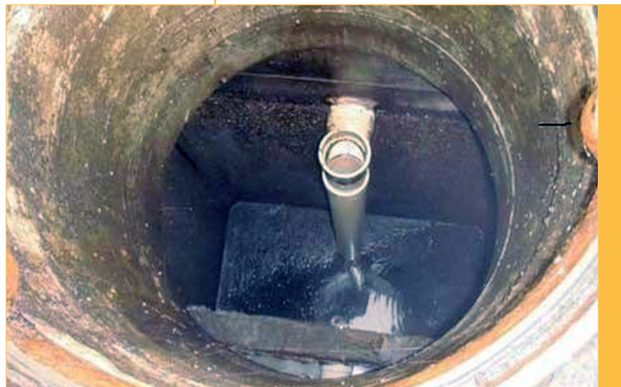
Gravity grease interceptor
