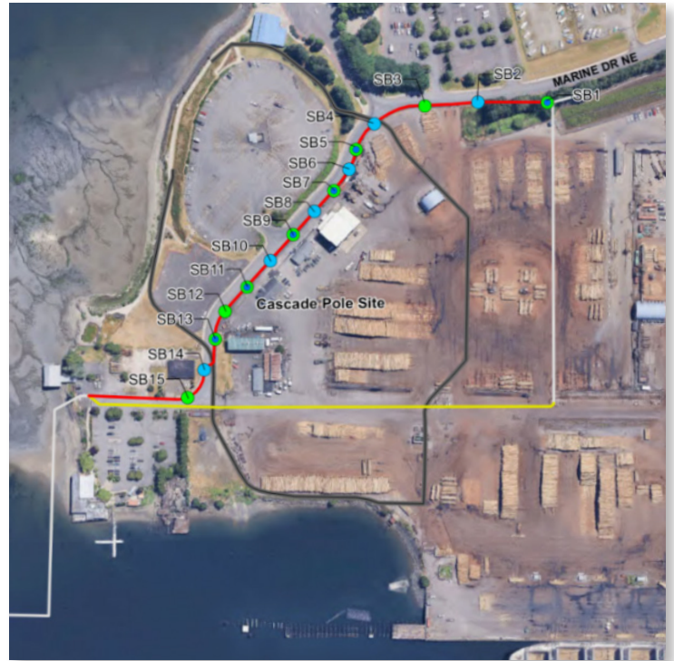
Aerial view of the North pipeline construction area.
